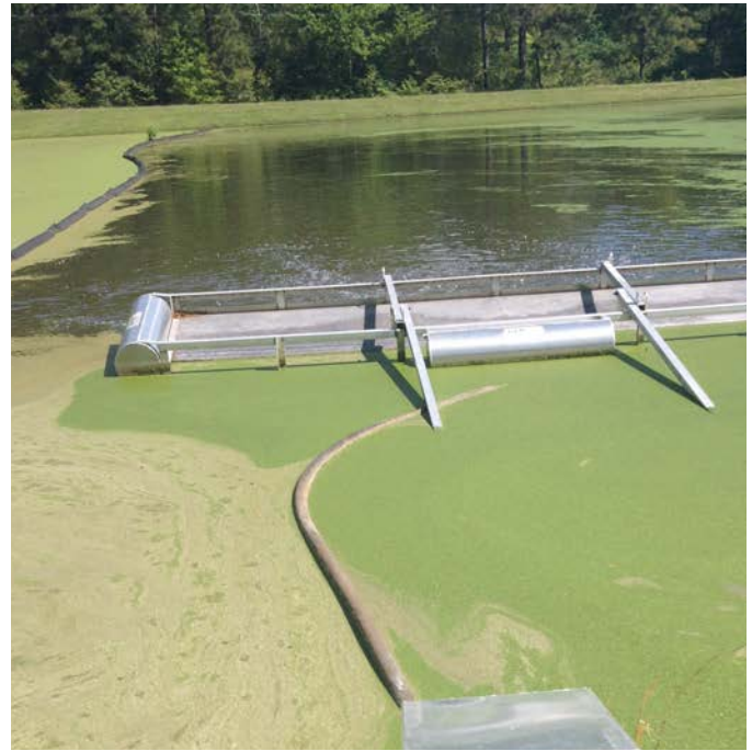
Lagoon Water Nitrification
