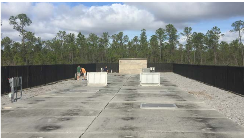
30,000 gallon decentralized system
